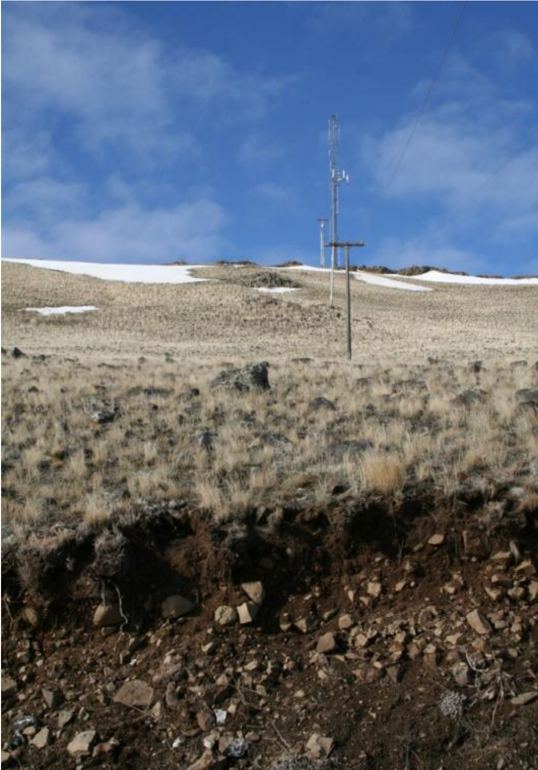
Figure A.43. Benton PUD Electrical Line (Locale 9B). Photo taken at 245 degrees on 3/20/09 by Doug McFarland.
