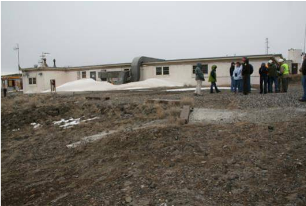
Figure A.6. View of 6652-C Building from the Ridge Edge Looking Up (Locale 3). Photo taken at 80 degrees on 3/19/09 by Doug McFarland.
