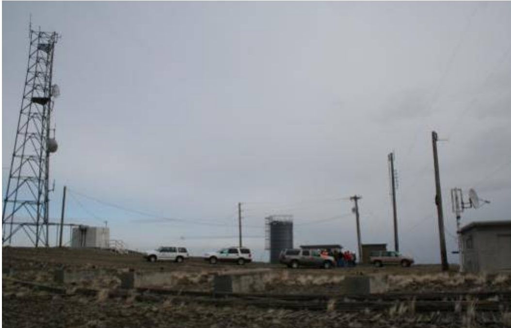
Figure A.8. Current Buildings and Proposed Location of the CCCF Structure and New Antenna (Locale 4). Photo taken at 20 degrees on 3/19/09 by Doug McFarland.
