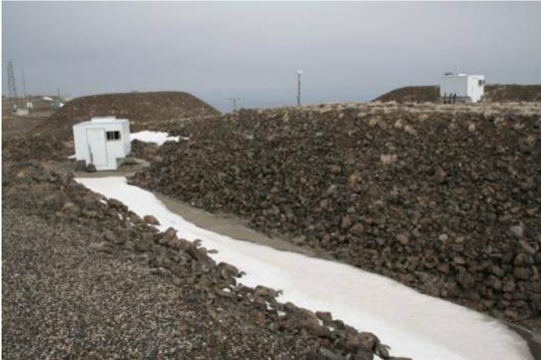
Figure A.1. Trailers Near the Observatory (Locale 3) to be Removed. Photo taken at 350 degrees on 3/19/09 by Doug McFarland.
