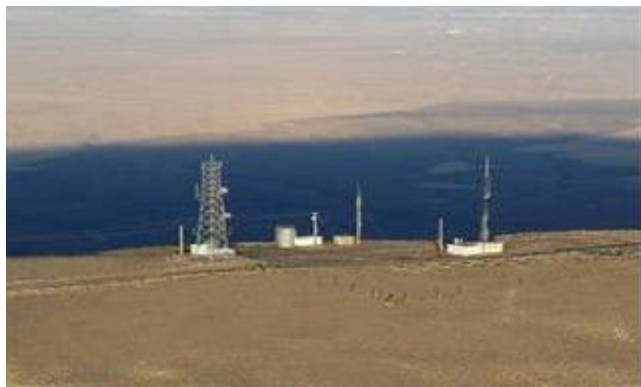
Figure 3.3. Energy Northwest Communications Site. The Energy Northwest lattice tower is on the left; all of the other facilities are proposed to be demolished.
