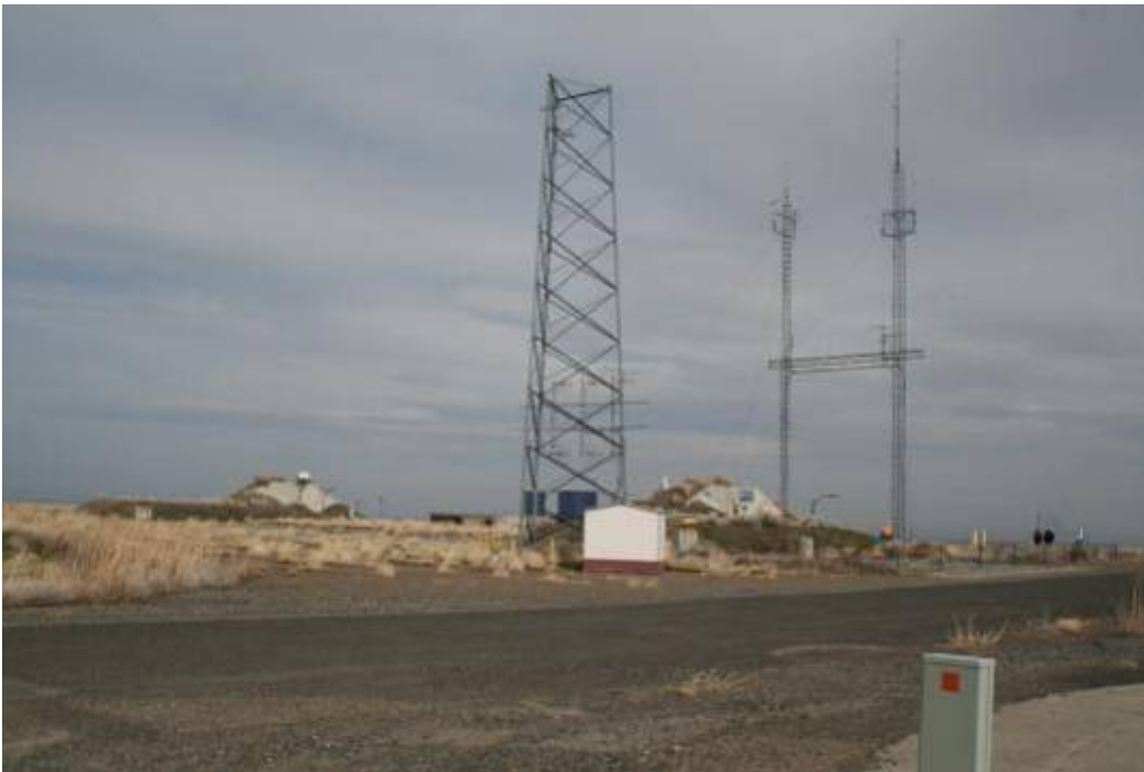
Figure A.34. Nike Bunkers and Radio Towers (Base Area). Photo taken at 20 degrees on 3/19/09 by Doug McFarland.
